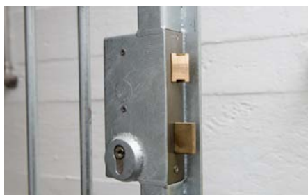
4 Locking on the side by means of brass spring bolt and bolt through use of lock case no. 140UMV.
