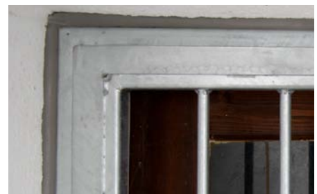
2 Stop strip on all sides of door leaf or door frame to make use of a pry bar more difficult.
