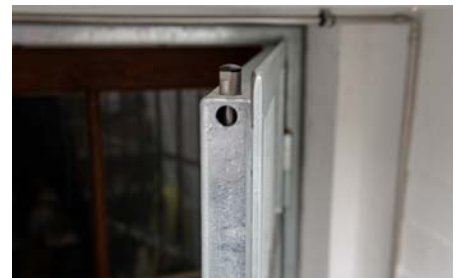
3 Locking at top and bottom through use of lock case no. 140UMV.
